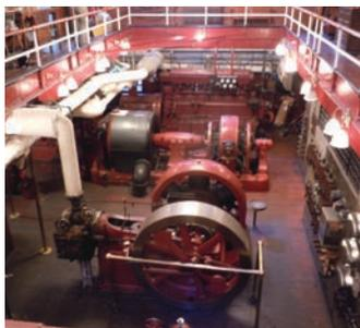
The plant provided power to the institute from 1887 through the 1970's. The oldest units are 3 reciprocating steam engines direct connected to dc generators installed in 1900. The engines can operate but the generators are disconnected.
