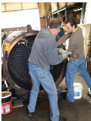
A worker stationed at one end would drive the tube out using a 2 foot long forked end special tool and a ten-pound sledge. Another worker would finish pulling the tube at the other end. Intensive labor with many rest periods ruled the day. Chris's crew made minor repairs to the tube sheets. The volunteers polished all 450 holes to insure proper fit for the new tubes and then loaded all the rest. Chris's crew trimmed
