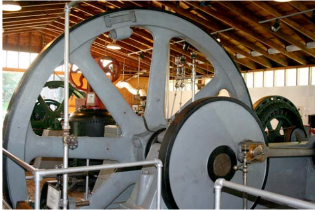
Figure 6 Bob (top) and bottom (Armington Sims Co., Providence, RI, steam engine, built in 1883) in the Steam Engine Heritage room.
